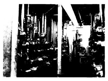
Six spiral heat exchangers were installed to cool the incoming juice and reheat the treated juice.
