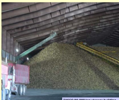
TASCO 80,000 ton storage building
