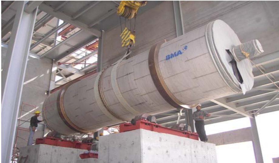
Fig. 1: Installation of a rotary dryer/cooler Ø 2.6 x 9 m
