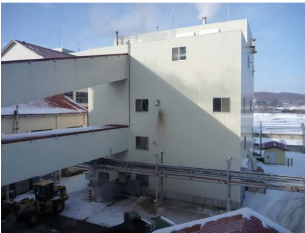
Fig. 2, steam dryer building at winter time.
