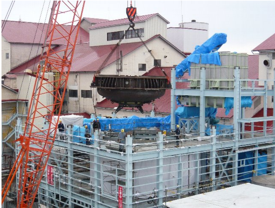
Fig. 1 The bottom part of the dryer is lifted in place.
