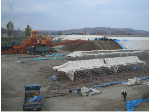
Fig. 6, beet piles are covered with tents.
