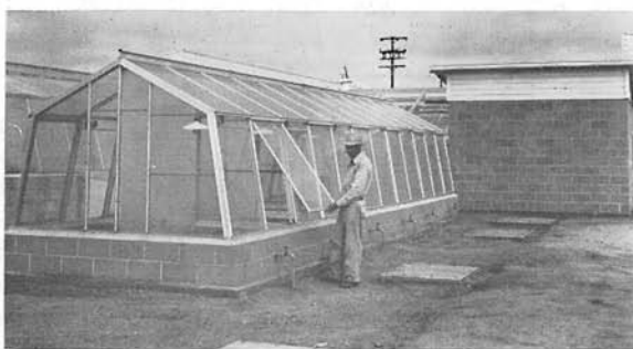
Figure 1.—Compartmented greenhouse used for production of sugar-beet seed at Salinas, California. Filtered air from fan house (top, right) is supplied to each chamber through underground ducts.
